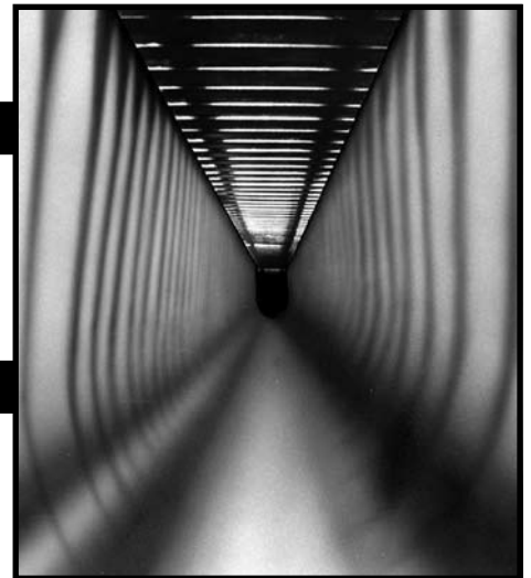
ABOVE - Smooth interior finish of drain assures complete drainage.
