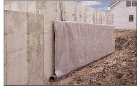
Residential & Commercial Foundations
